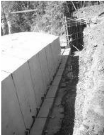
29 TON ARCH BEING SET IN PLACE
