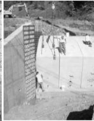
29 TON ARCH BEING SET IN PLACE
