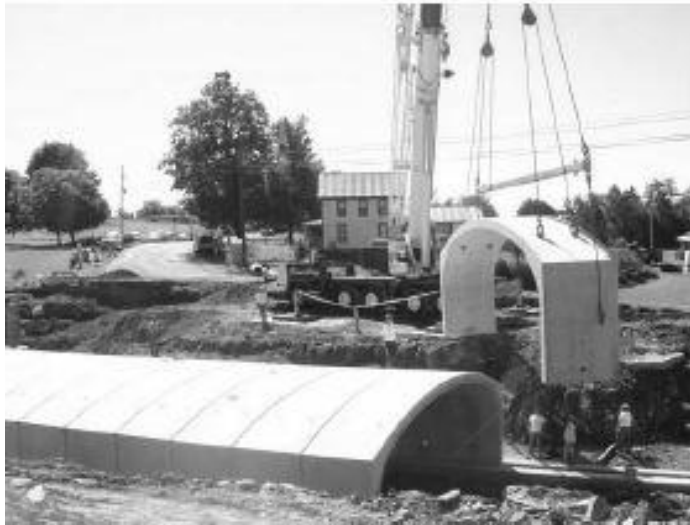
29 TON ARCH BEING SET IN PLACE
