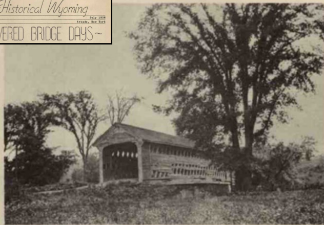
Ellis-Chesbro Bridge, Bennington, The Last Covered Bridge in Western New York. (Photo taken c1926 by Mrs. Elise C. Emt.)
