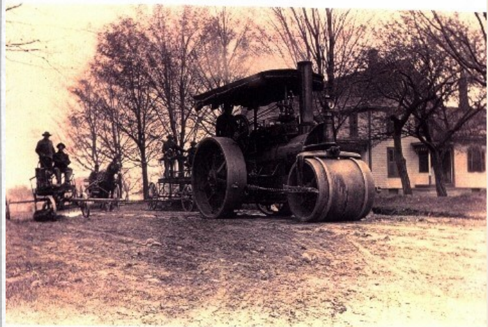
Steam tractor grading the road in front of the John Dominesey homestead, on Route 77, between Perry Rd. and Sheldon Center, about 1910.
