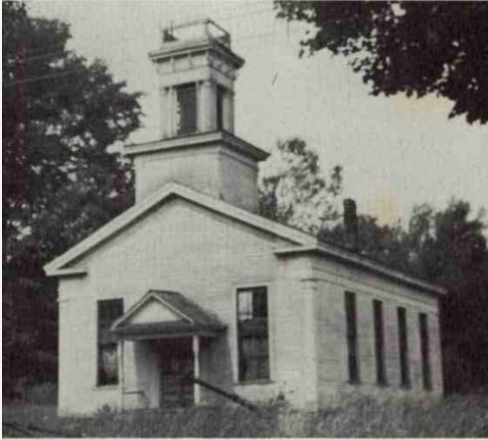
Johnsonburg Presbyterian Church Erected in 1858
